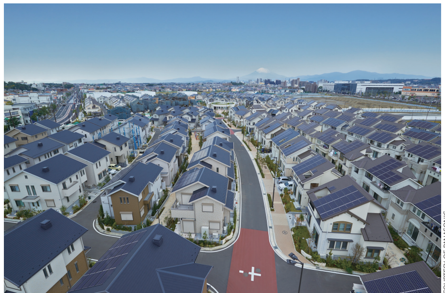
Fujisawa Sustainable Smart Town (Fujisawa SST) in Fujisawa City, Kanagawa Prefecture
