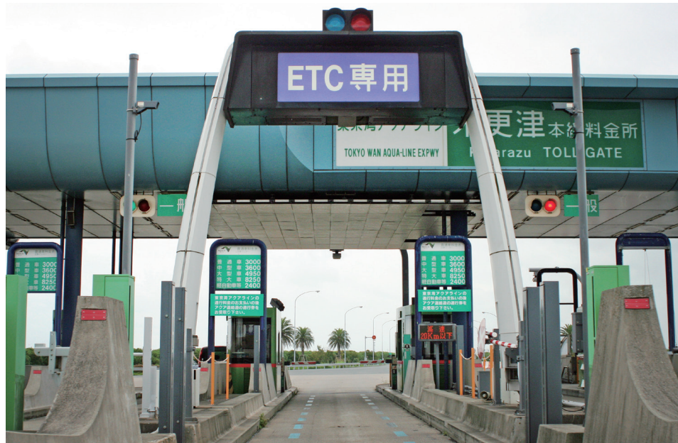
An ETC tollbooth on the Tokyo Wan Aqua-Line Expressway. The ETC (electronic toll collection) system has significantly eased traffic congestion at tollbooths on Japan's expressways and allowed for more flexible pricing.
