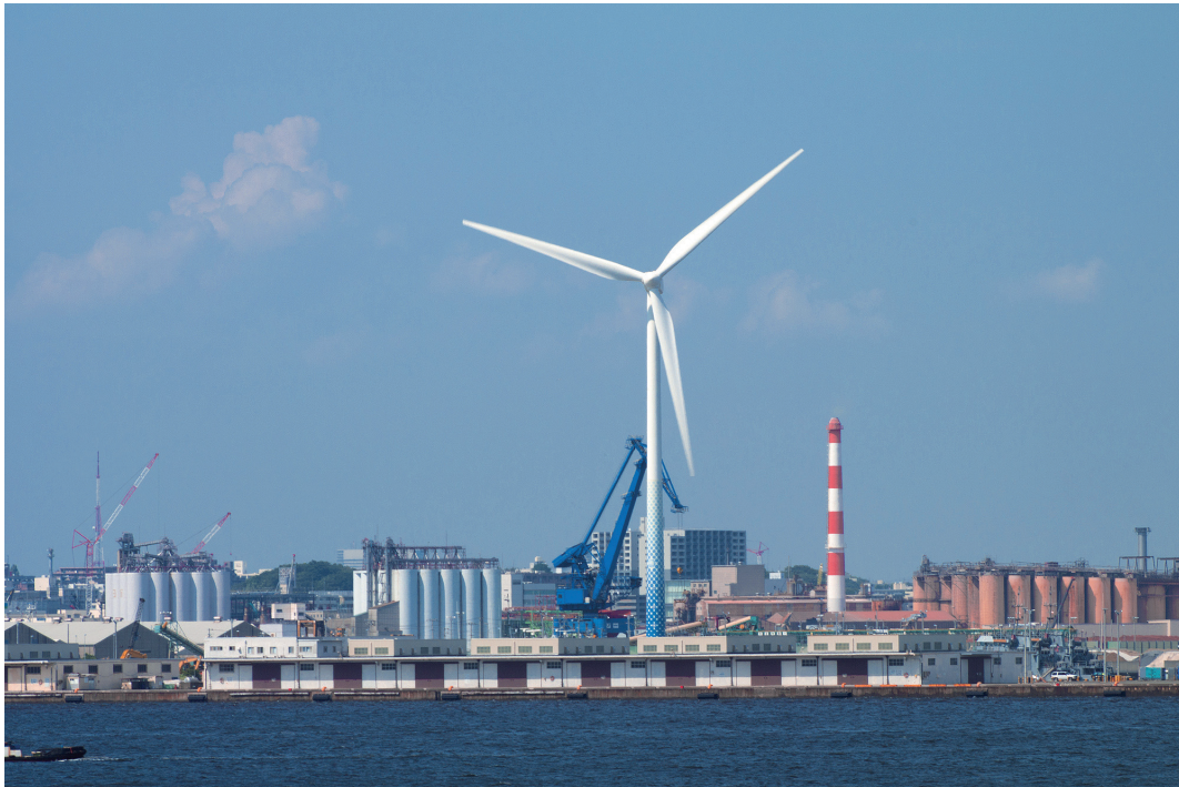
Hama Wing, the experimental wind power plant in Yokohama, Kanagawa Prefecture
