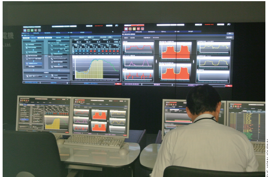
Monitors in a community energy management system (CEMS) operations room in Higashida Ward, Kitakyushu, Fukuoka Prefecture display graphs and figures showing electric power supply and demand.
